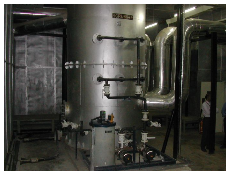
Image 1 - Scrubber for DG set during Installation
