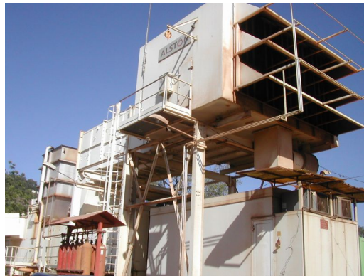
Air Intake System for MAN DG set 1.9 MW for Sudan GT Air Intake system 5 MW unit for Alstom Turbine at Maali
