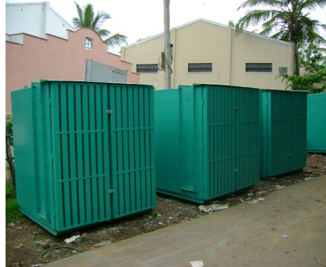
Air Filtration Unit for 2 MW DG Set for MTU France Thru Angelique to Rep of Maali
