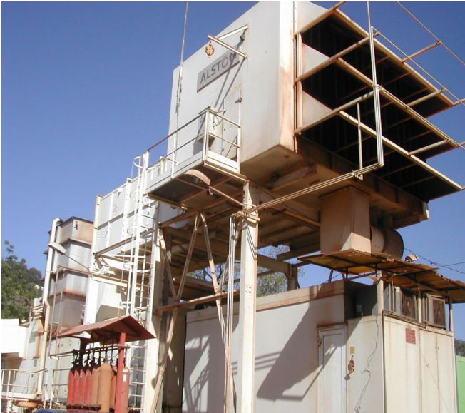
8 MW G.T Air filtration, acoustic and Exhaust Silencers at Bamako (Rep Of Maali) Africa.
