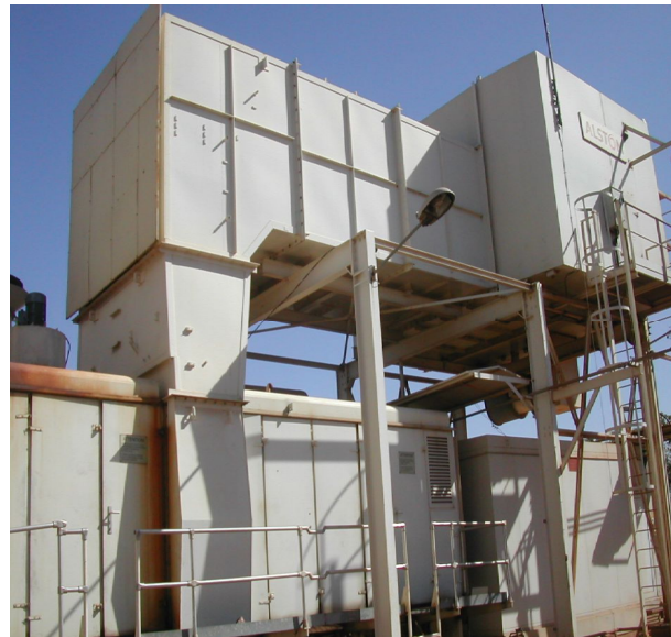
8 MW G.T Air filtration, acoustic and Exhaust Silencers at Bamako (Rep Of Maali) Africa.
